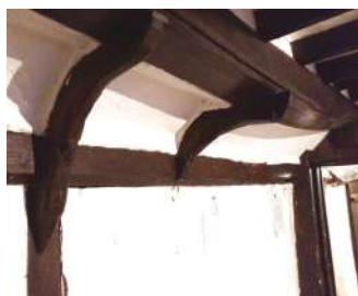
Left: Probably re-used ship's knee braces in the Mint House. Right: Knee Brace in a ship at the Shipwreck Museum in Hastings. Photos: Lisa Fisher
