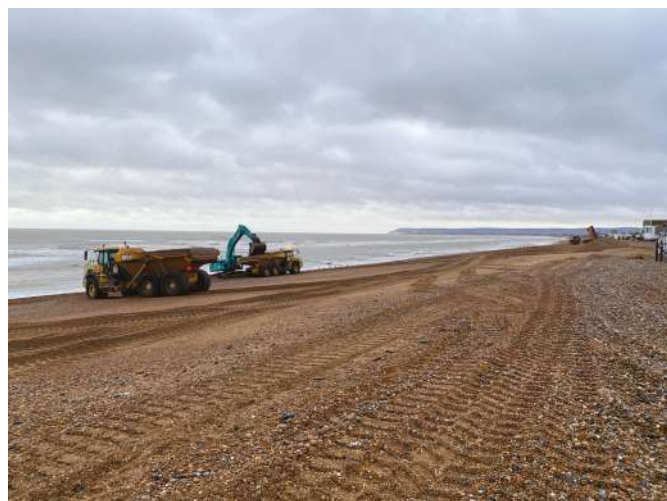
Storm Goretti recovery works on Pevensey beach, 9th January, 2026
