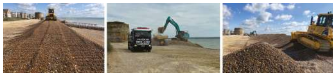
Beach replenishment works using recycled shingle from the Hastings trial
