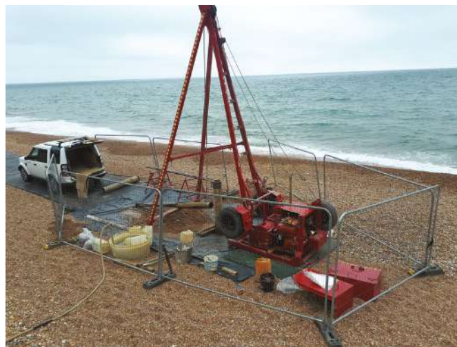
Typical set-up for ground investigations, including drilling equipment and temporary safety fencing
